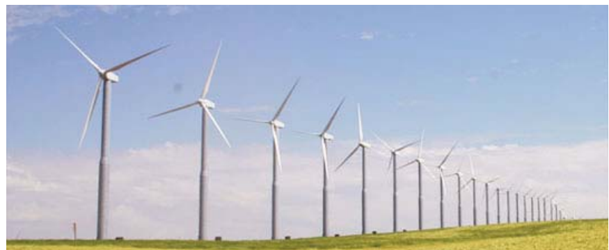
Much of Whitman's power through the Blue Sky program comes through wind turbines. Whitman recently increased the amount of wind energy it buys from 180,000 to 2,202,000 kilowatts per month
